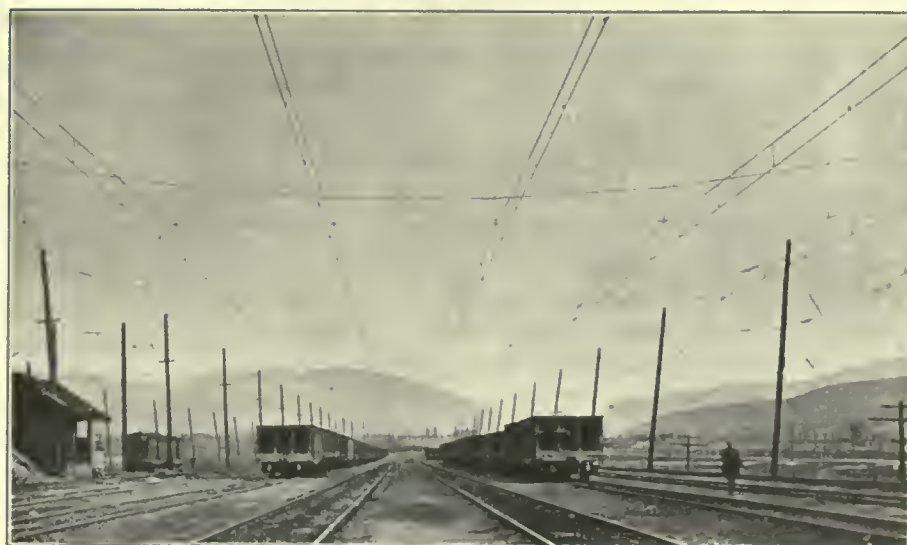
FIG. 530. OVERHEAD CONTACT SYSTEMS. Single Catenary 2,400-Volt Direct Current Yard Track Construction, Butte, Anaconda & Pacific Railway.
